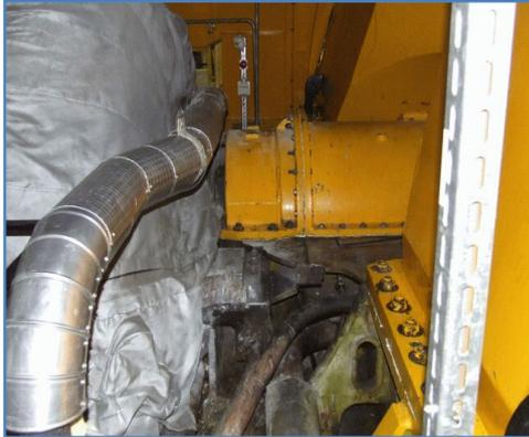
**Assessment:** The self-ignition temperature of oil is 390 °C. This temperature level was surely not reached on the spot. The „Rockwool” isolation material, which was present at the oil spot, reduced the flashpoint of oil. The isolation material is supposed to have absorbed oil which had filtrated through the minor leakiness and after turbine heat up a self-ignition occurred.
