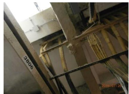
*Picture 3: Fire barrier wall penetration*
