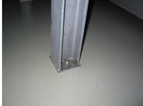
*Bolted joint on the filter frame foot*
